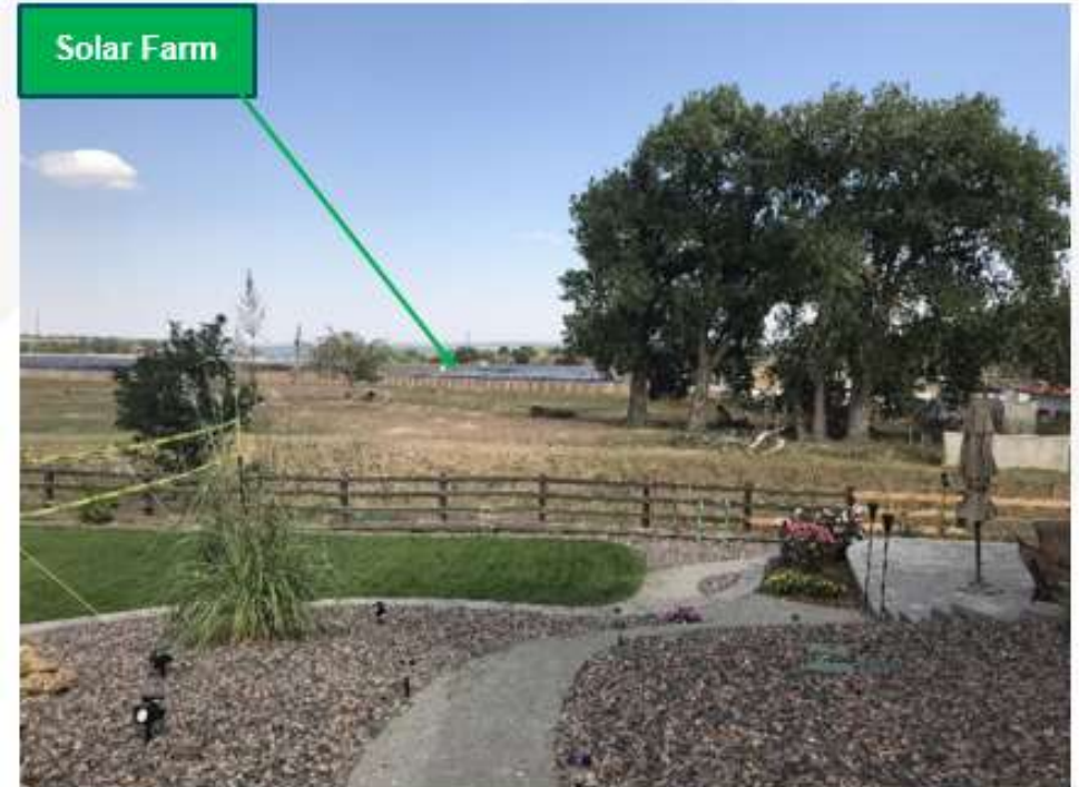
View from the Rear of a Test Area Home, towards Solar Farm
